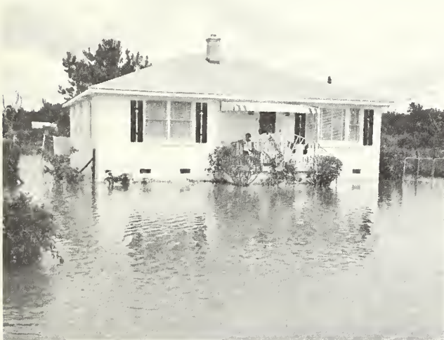
FLOODED SUBDIVISION - With disruption of utilities and property damage.
